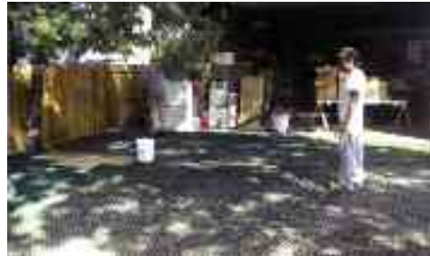
BodPave®85 porous grids during installation
