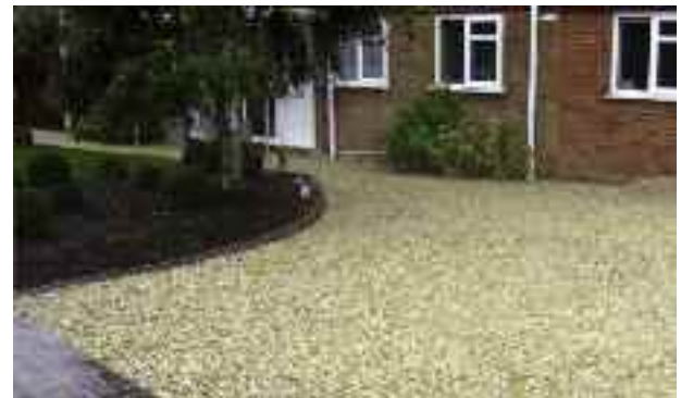
Filled with angular gravel creating an attractive reinforced permeable surface that retains the gravel
