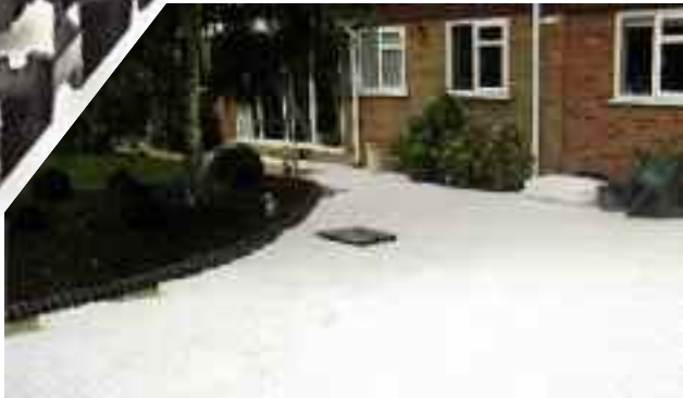
BodPave®85 natural (white) pavers installed for a domestic driveway application
