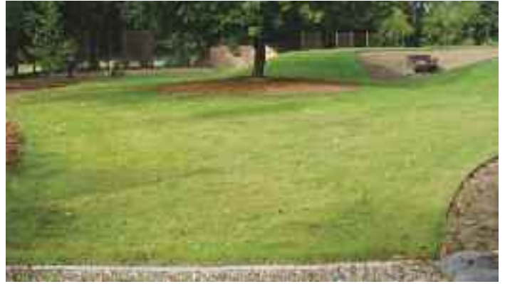
After just a few weeks... the grass grows through the mesh offering a strong stabilized surface.
