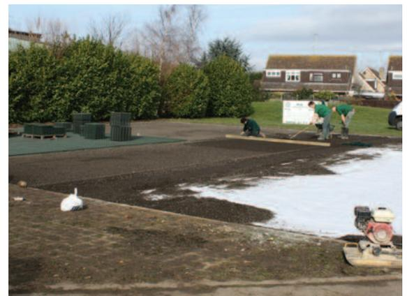
Typar 3401 geotextile fabric installed within a BodPave® porous paving construction
